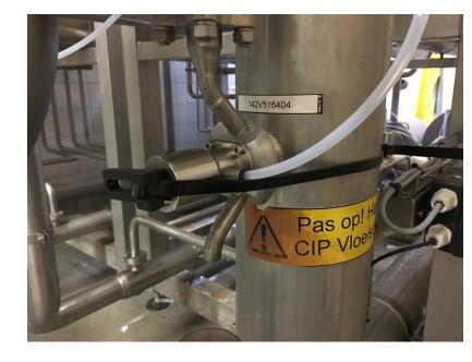
contamination. The folds of RIEGER's PTFE bellows always stay open during cleaning and allow all product remainings to be cleaned out. The PTFE bellow of the BioCheck Valves is optimized even more and only has one fold. Metal bellows have their folds moving together completely, so product can get trapped and stay as a potential growth area for bacteria within the product touched surfaces.
