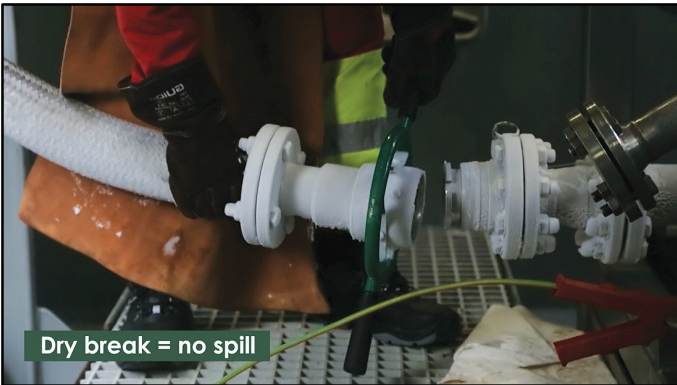
Disconnecting 3" Cryogenic Hose
